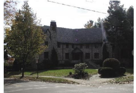
The Chi Phi house will be undergoing renovations, possibly as early as this summer.
