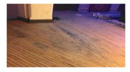
This is a recent photo of the existing hardwood flooring installed in 1932. Refinishing over the years has opened up the joints between each board to a point where re-sanding and refinishing again is not an option. Don't you wish your floors lasted for 85 years!
